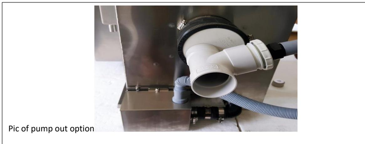
The pump out option enables users to occasionally empty and flush out the unit. (You may want to do this to eliminate odour build up). It may also reduce the frequency of external pump outs.
